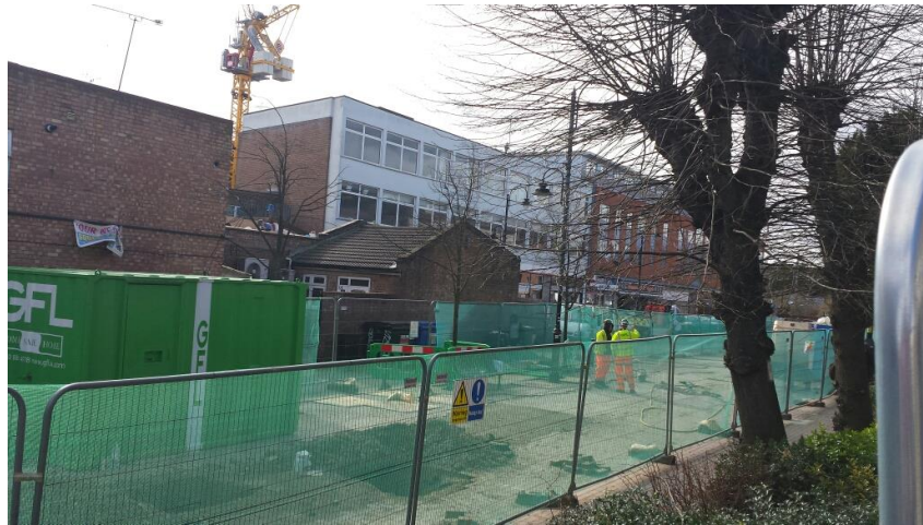
Works at Wealdstone Square
